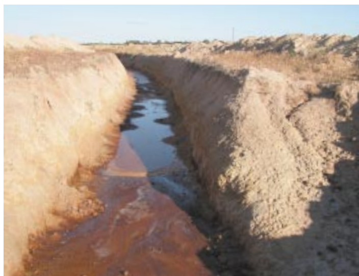
Iron precipitates in drain base, source of acidity
